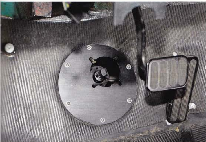
14. A new plate may be needed if the previous one was adapted for the offset column location. Here, a new plate has been installed; note the relationship of the steering shaft with the column opening.
