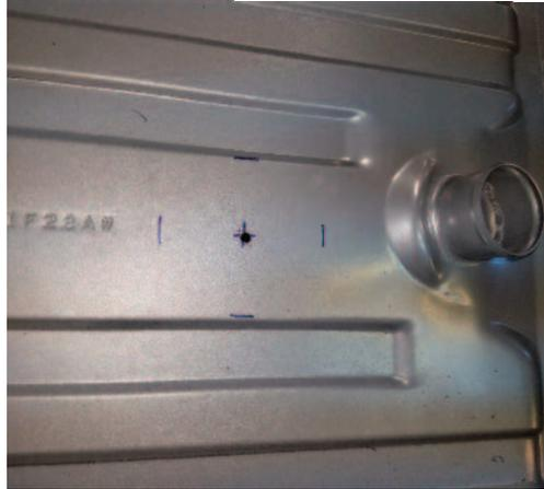
7 Then cut a 4 1/2" hole using a 4 1/2" hole saw with a slow speed drill.
