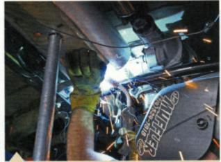
Now the head pipe gets MIG-welded to the inlet of the 50 Series SUV muffler for good! In tight spaces, you can cut back the inlet and outlet tubes on the mufflers for more tube clearance. Make sure to wear proper welding gear if you are pulling the trigger.
