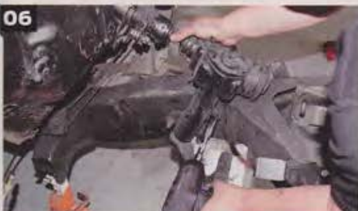
06. We removed the through bolts that hold the steering box in place on the frame. This can be a bit tricky to do with the engine in the way. The best tip we can offer is to remove the driver's side exhaust manifold or header for access.
