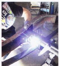
With the angles set, the pads can be welded. Ultimately, if you're fully welding the spring pads to the housing, warpage caused by heat is more than likely, thus the importance of having the housing straightened (or at the very least checked for straightness) afterward. For the time being, we put 3/4-inch welds at each corner of the pads.
