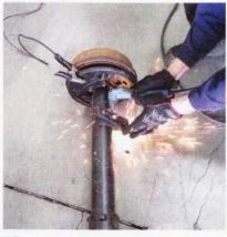
16... And since the Miller 375 xTreme was already warmed up, we also plasma-cut the existing spring pads off the 10-bolt, leaving just enough to smooth off with a grinder while not getting too close to the axle tubes to cause any warping.
