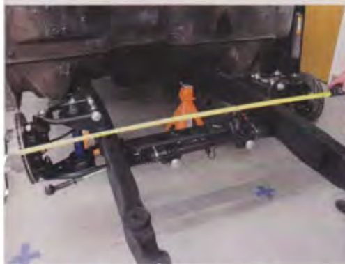
129. With the rack in place, it's time to hook up the outer tie-rod ends to the spindles. I typically set up a new front end with \frac{1}{8} -inch toe in, which is what I'm doing here.
