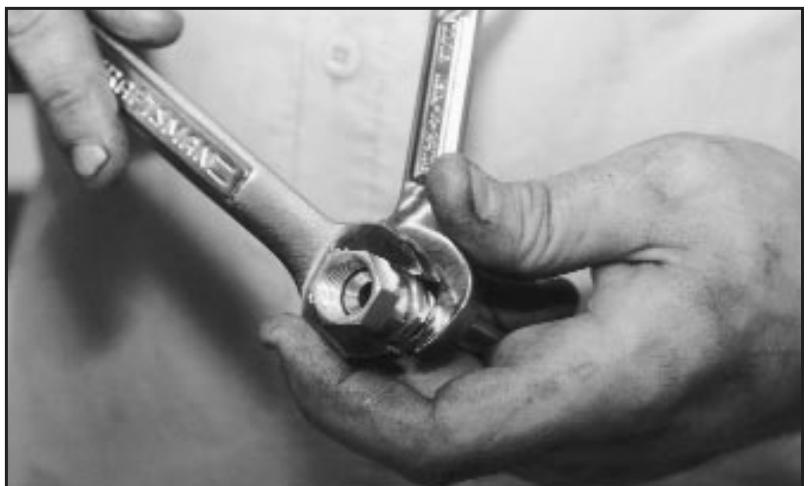
**Once the pieces seated, he tightened them with two wrenches. Yet an easier way would be to hold the fitting's collar in a vise and tighten the nipple portion with a wrench.**
